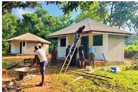
(right) renovation of two 'Bandas' at the Buwenda Scout Campsite
