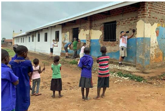
(left) refurbishing school classrooms
