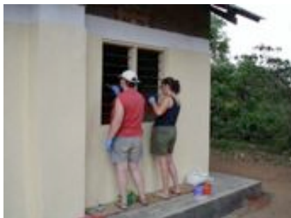
Refurbish school classrooms at the Kavule School for the Deaf, Mbale
